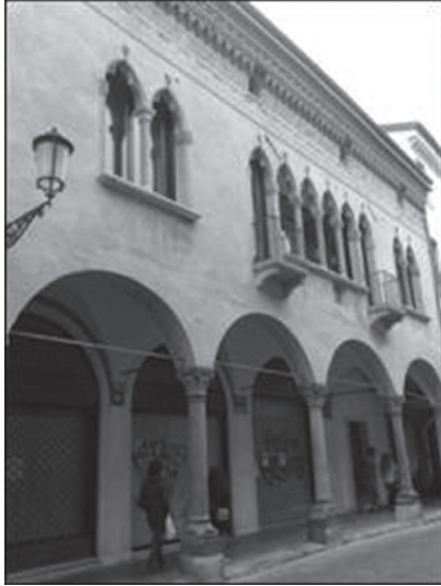
Fig. 9. The Pinelli House in Padua (known as Casa Casale, Via del Santo 127-131)
